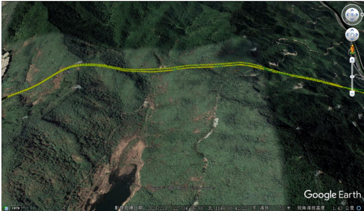
横龙山隧道/Henglongshan Tunnel
